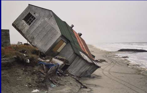
Figure: Melting Ground and Sea Ice Destroying Villages in Alaska, Source: globalwarming.house.gov
