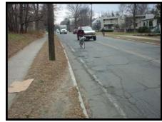
shoulder is the worst contiguous road surface of all the links discussed here. Bicycle travelers are forced to follow an inconsistent path, moving further than acceptable into the vehicle lane and to be extremely careful with bike handling. There are also very high volumes of car and bus traffic on this link as it is the main connector to the Amherst downtown area and areas southeast of campus.
