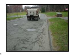
surface is very broken, uneven, and there are many potholes and manhole covers that break up the line of travel. Combined with the grade of the road, the commuter who is descending the hill must be very comfortable with bike handling, braking, and riding in traffic in order to safely navigate their way into campus. Construction vehicle traffic is also very high on this route and near the Sylvan dormitories the road is not wide enough to accommodate a cyclist and dump truck in the same lane.
