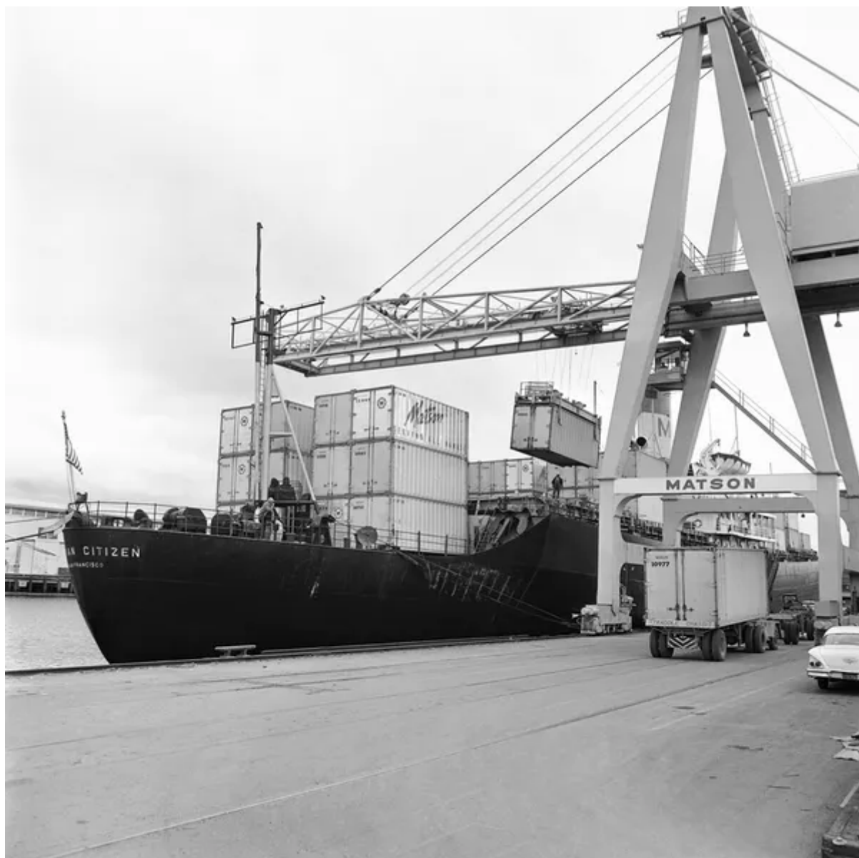
The Matson Hawaiian Citizen was one of the first ships converted into a container vessel, seen here at a San Francisco pier in 1963. AP Photo
